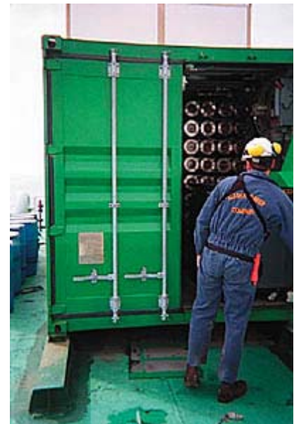
A BP Amoco PLC worker checks on a device designed to destroy foreign marine species in the ballast water of the company's oil tanker Tonsina.
